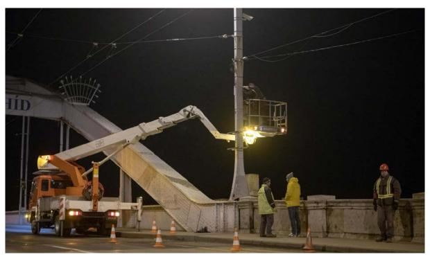
Installing the prototype of traffic data collection sensor
