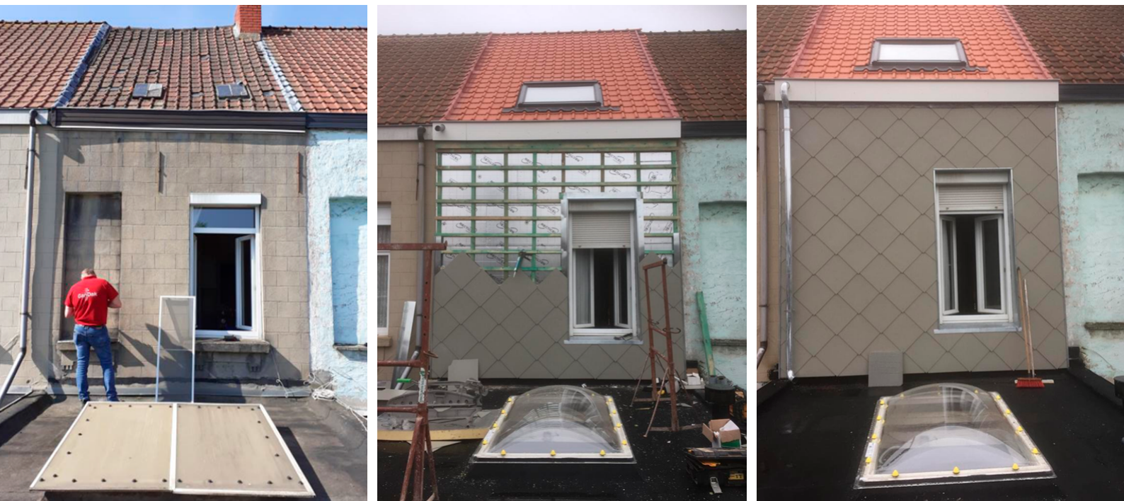
Image: before, during and after the renovations works. Here was focussed on renewal and insulation of flat and main roof, insulation of the back façade and a new skylight.
